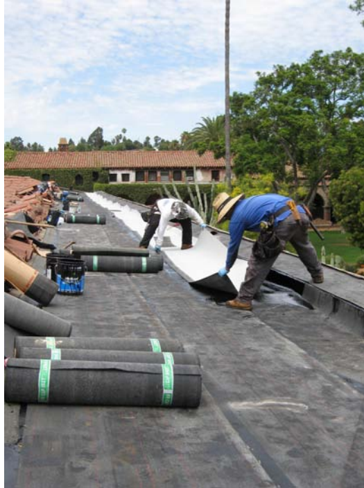
During Installation Installation of waterproof roof membrane
