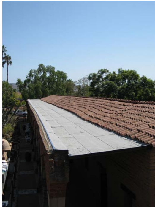
After Project completed.
