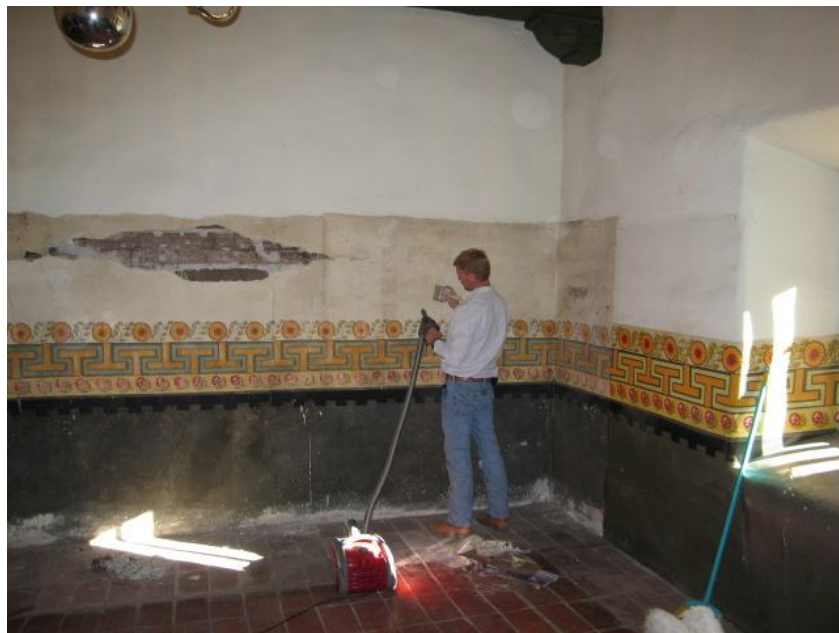
Sacristy after cabinet removal, note original decorative dado circa 1940s. November 3, 2008
