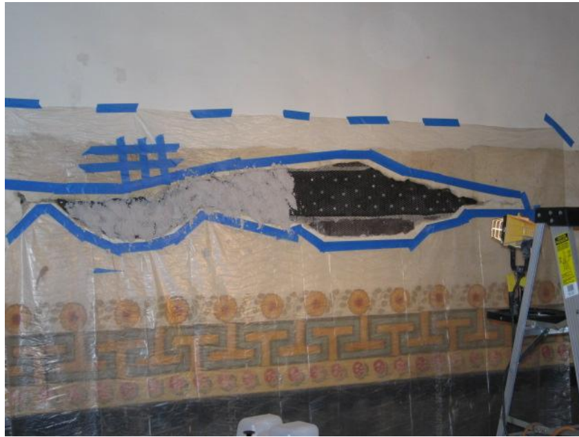
Plaster repairs prior to cabinet installation. November 10, 2008
