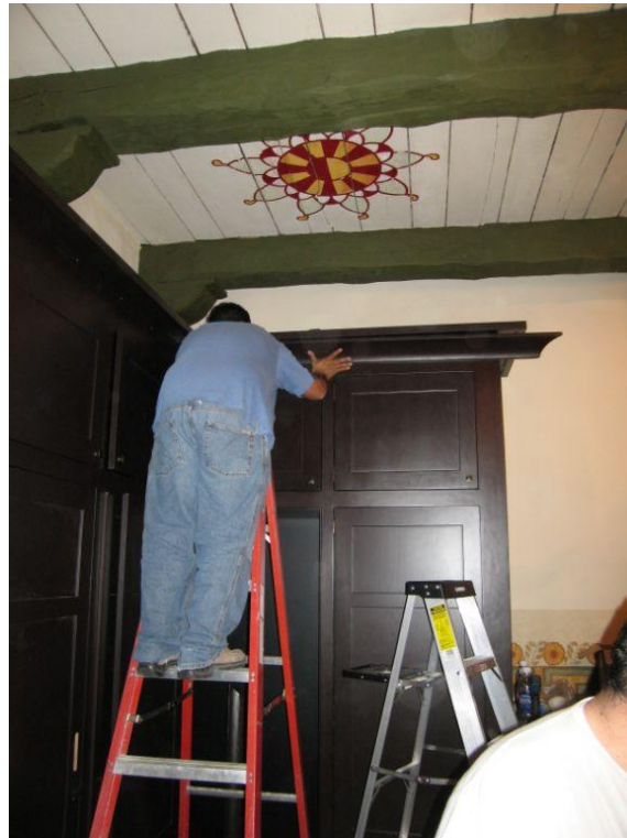
Installation of Sacristy cabinet finish details. December 16, 2008
