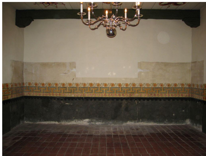
Plaster repairs complete, non-decorative areas of walls and ceilings painted. December 1, 2008
