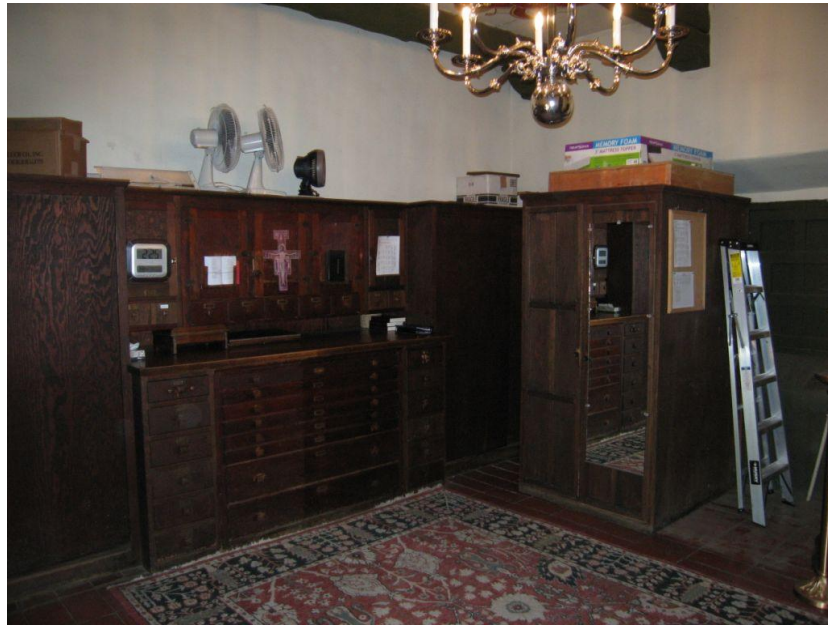
Existing Sacristy conditions prior to project start. October 27, 2008
