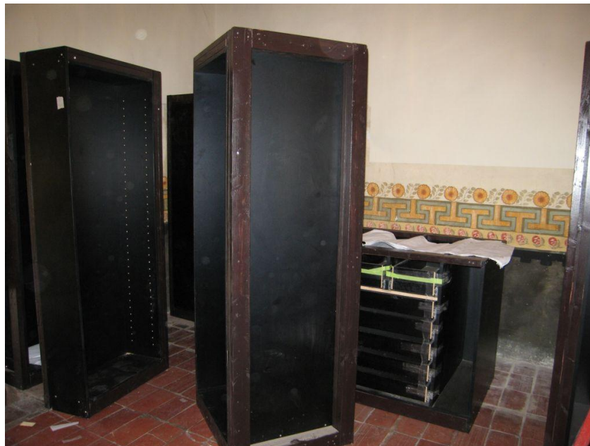
Installation of Sacristy cabinets. December 9, 2008
