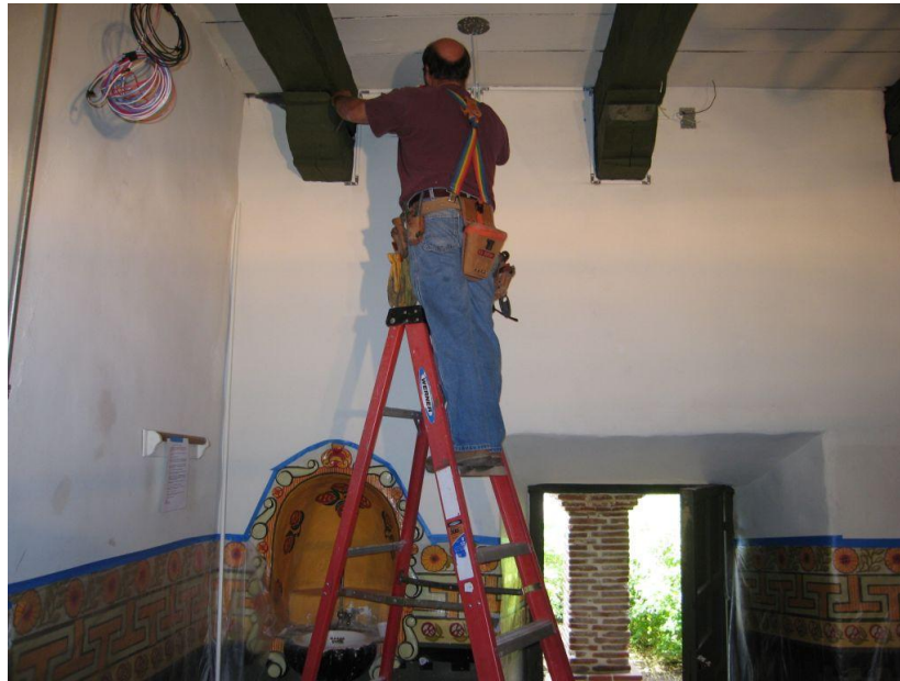
Installation of new electrical systems. November 17, 2008
