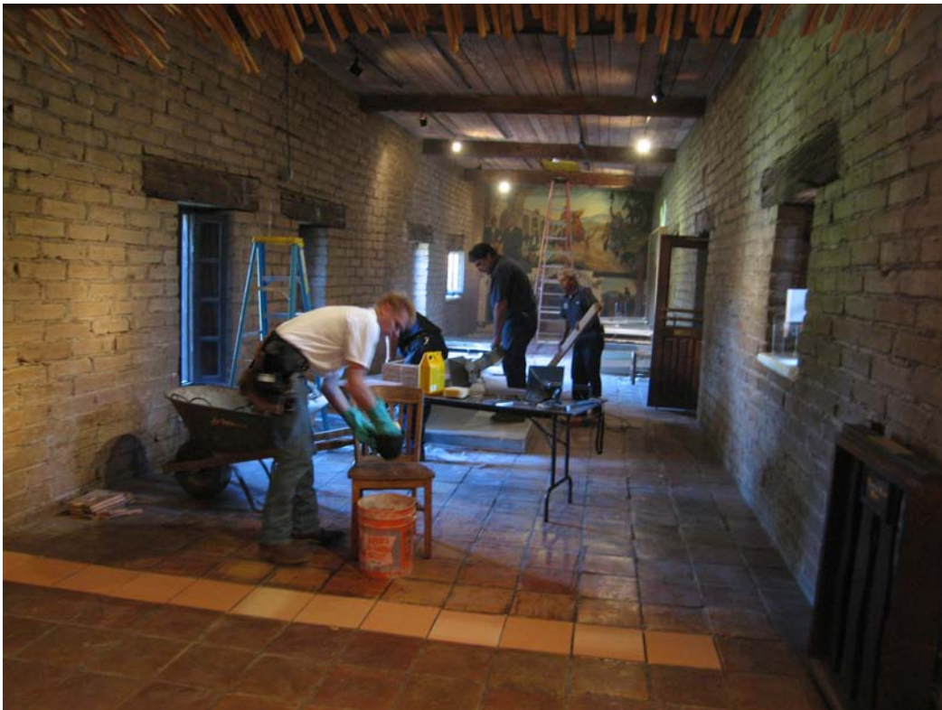
Repair of tile floor.
