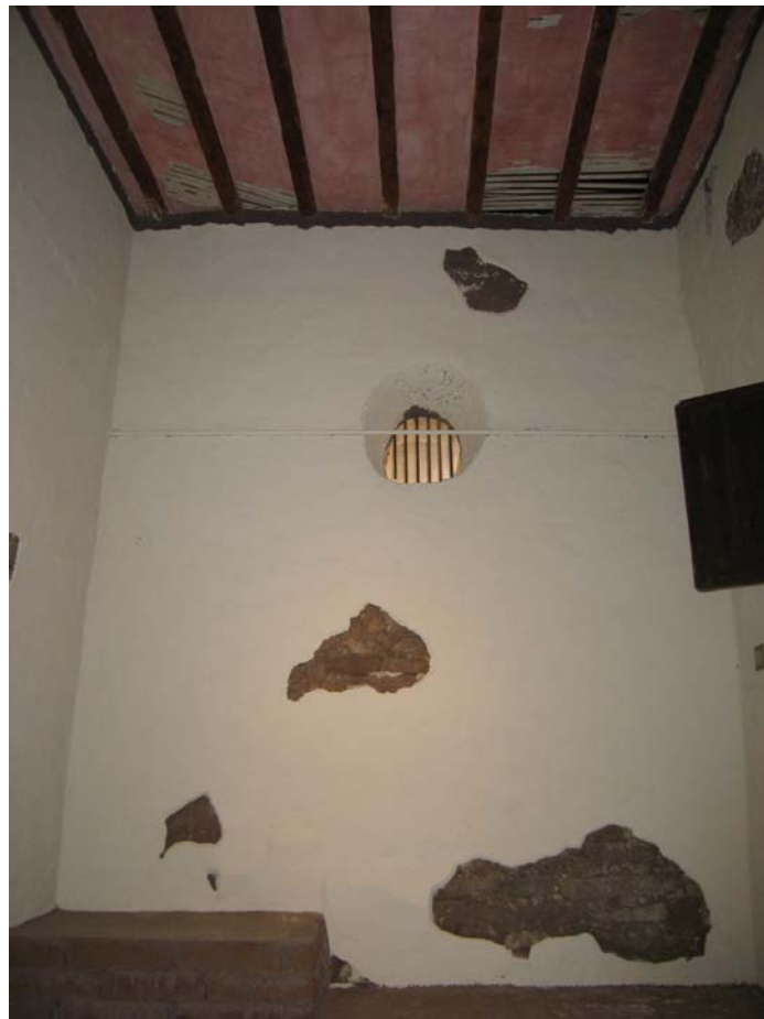
After Southern Dormitory wall after treatment
